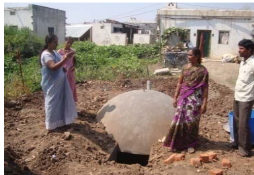
Bio-gas Plants Construction In Collaboration With NEDCAP
